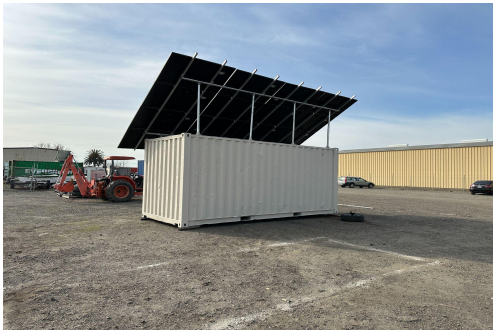
HEAVY DUTY CUSTOM PANEL INSTALLATION
